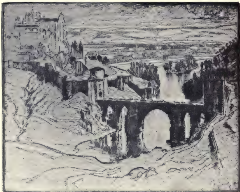
ST. MARTIN'S BRIDGE, TOLEDO Size of the original print, 7\frac{7}{8} by 10 inches. From the etchings by Joseph Pennell.
